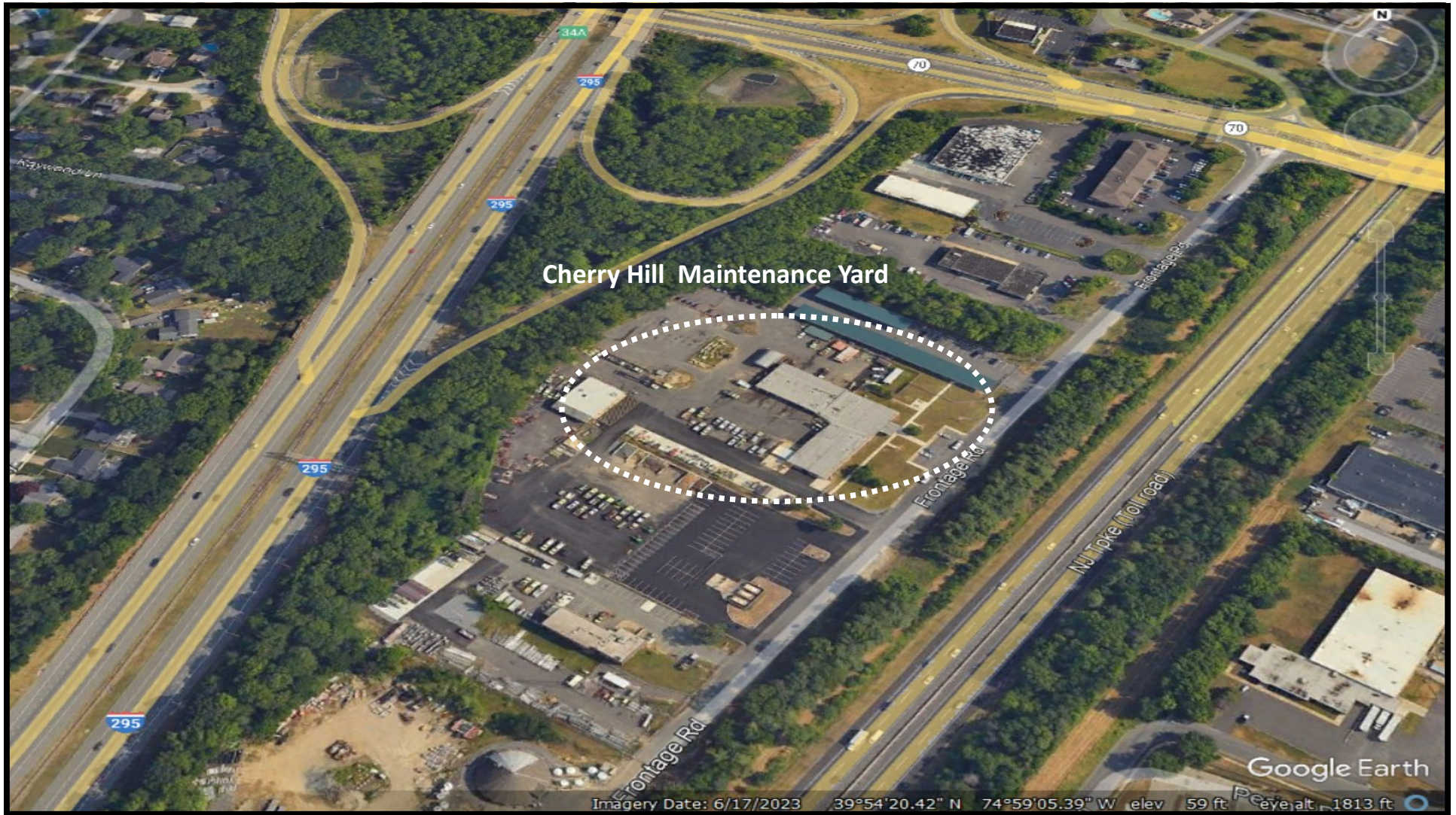
Project Location - NJDOT South Cherry Hill Maintenance Yard - Office & Garage Building EXHIBIT 'B'
