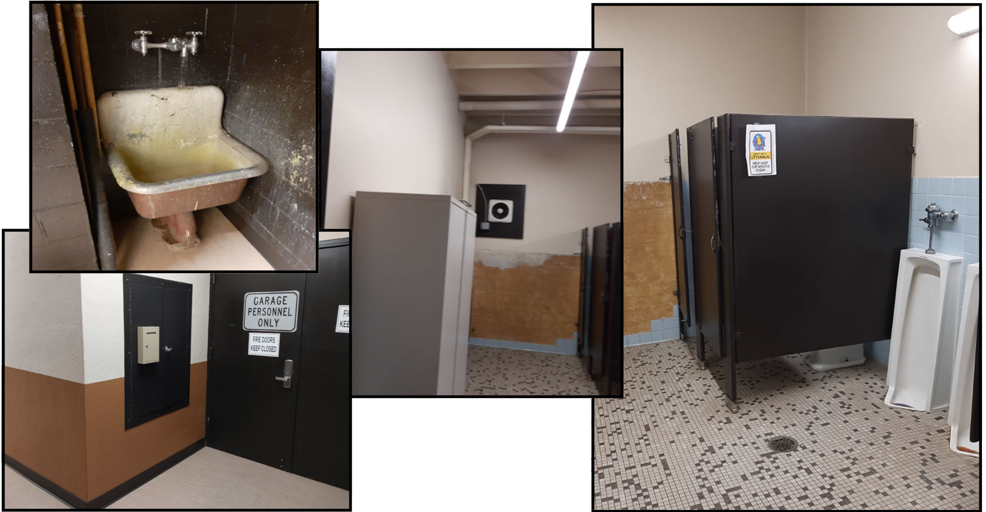
Photos - Garage/ Yard Area
