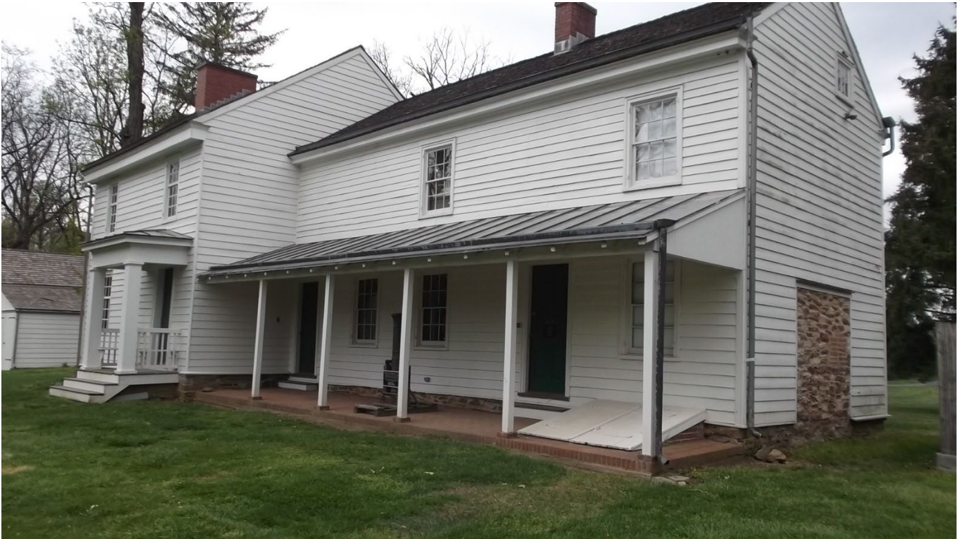
Clarke House at Princeton Battlefield State Park. An ADA accessible pathway will be required in this area. Carriage Barn in background to the left.
