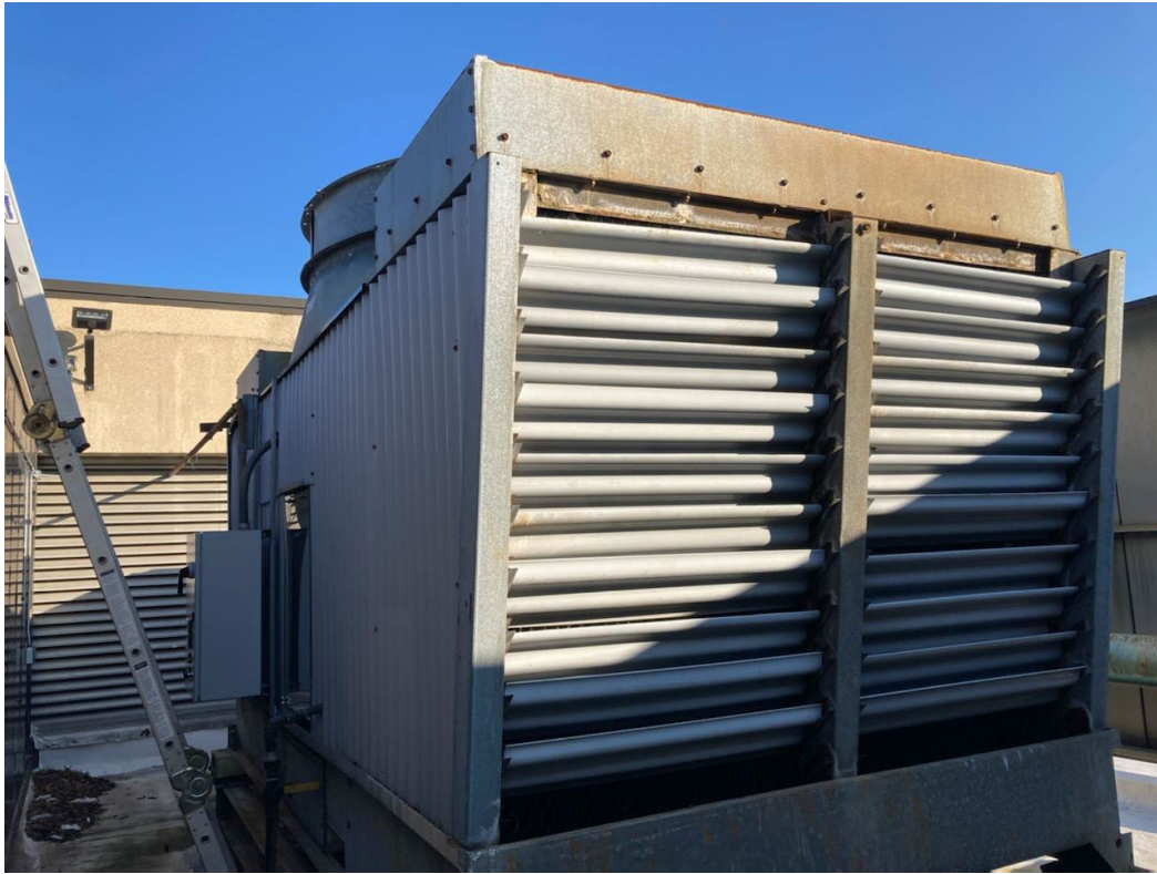
Cooling tower to be replaced.
